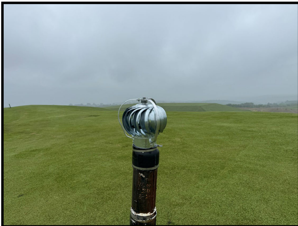
Photograph 4: View of repaired turbine vent on north side of Area 1-2.
